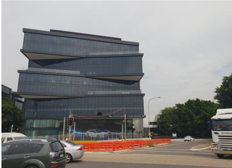
Figure 10. 185-1896 O’Riordan Street Mascot which is opposite the site
