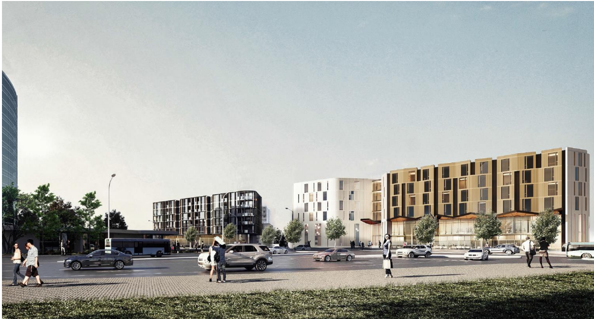
Figure 18. Perspective of the site viewed from the western side of O'Riordan Street
