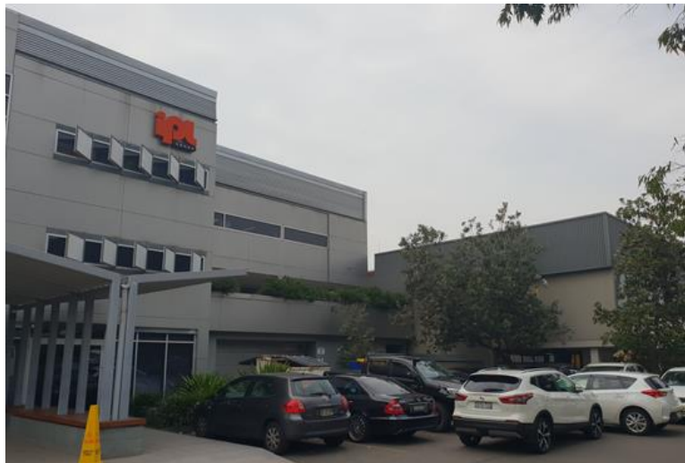
Figure 4. 146 O'Riordan Street (front elevation along O'Riordan Street)
