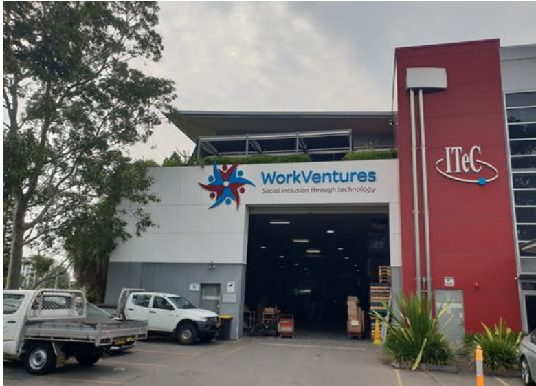
Figure 3. 146 O'Riordan Street (front elevation along O'Riordan Street)
